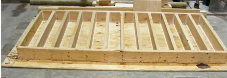
**FIG. 1. Beam formwork**
